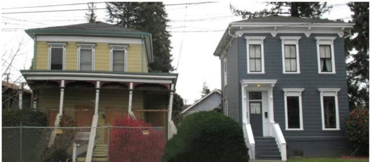
Unretrofitted and Uninhabitable
